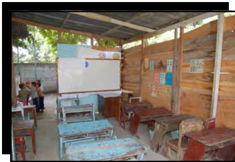
Existing classroom conditions
