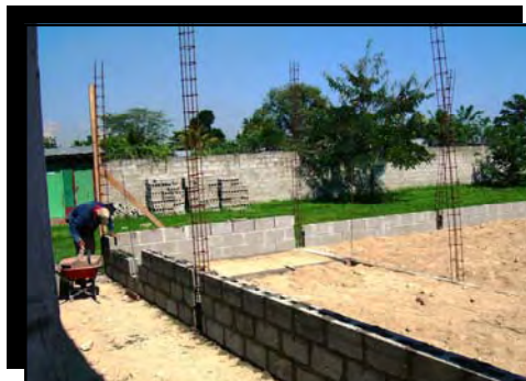
New school construction site
